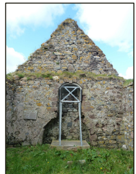
VIEW ON THE WEST GABLE OF WEST CHAPEL PRIOR TO PHASE 1 CONSERVATION – METAL SUPPORTING SYSTEM WAS LATER REMOVED
