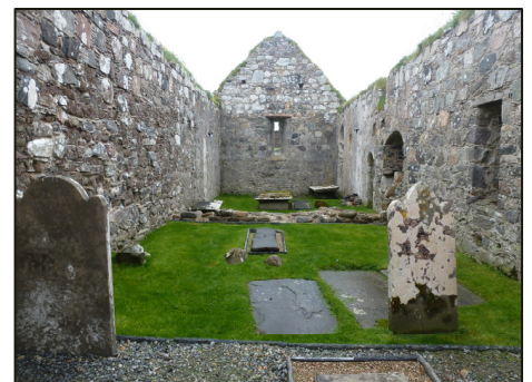
COMPLETE WORKS AT THE CHURCH VIEW TOWARDS EAST
