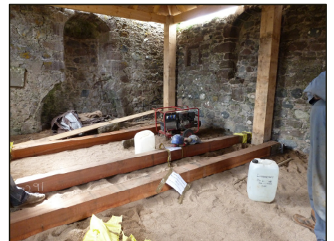
INSTALLATION OF TIE/STRUTS SYSTEM AT WEST CHAPEL
