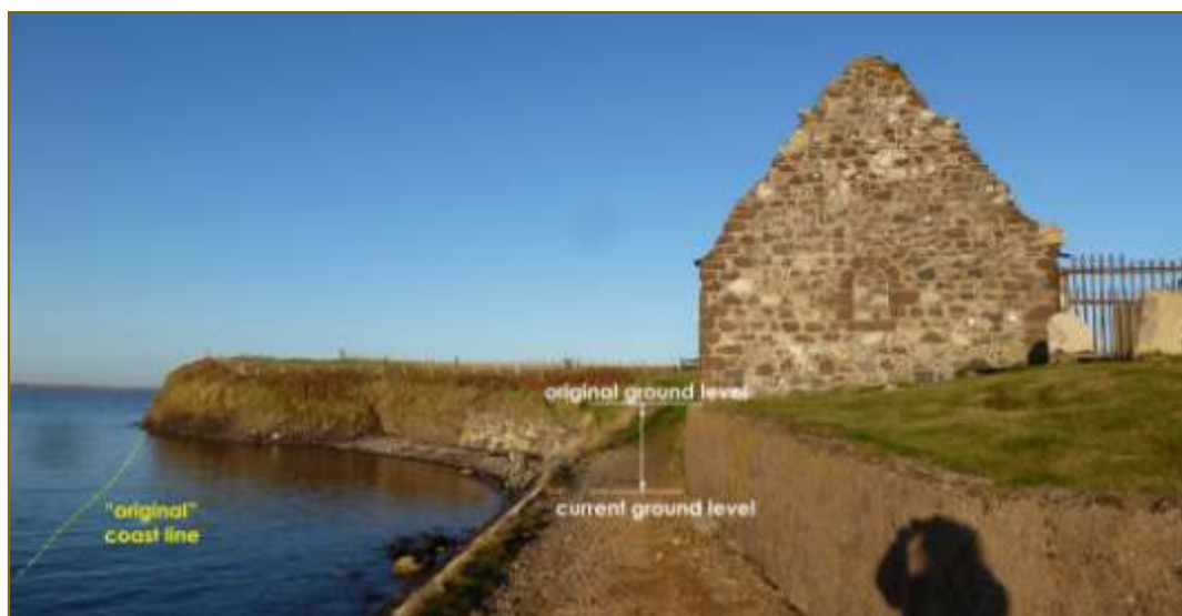
COASTLINE EROSION SHOWING EXTEND OF LAND LOST TO SEA
