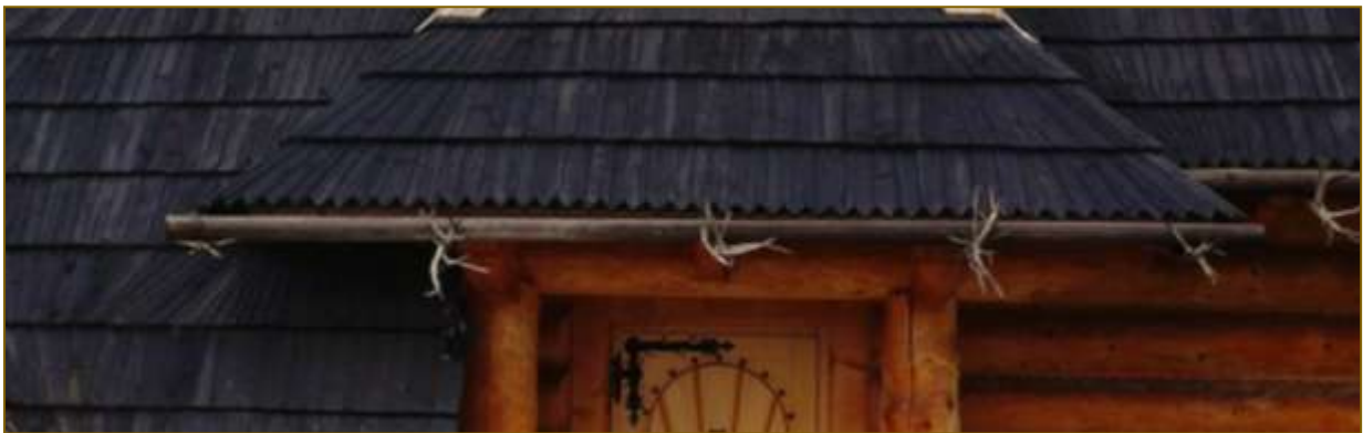
EXAMPLE OF SHINGLE ROOF WITH WOODEN GUTTERS
