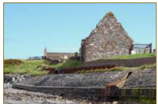
VIEW FROM THE WEST - NOTE ROW OF SHEET PILES ALONG THE SEA LINE
