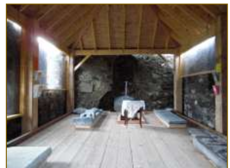
WEST CHAPEL WITH ITS TEMPORARY ROOF PROTECTING SLABS OF RODERICK MACLEOD (TOP LEFT) AND MARGARET MACKINNON (TOP RIGHT)
