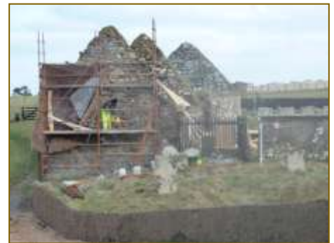
CONSERVATION OF WEST GABLE
