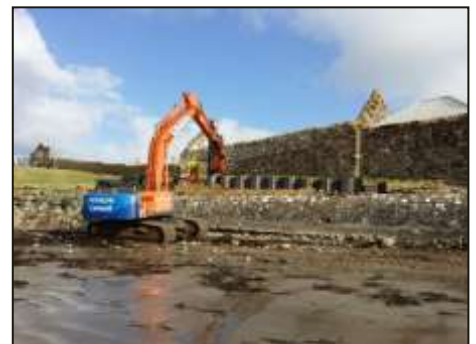
INSTALLATION OF SHEET PILES ALONG THE MOST VULNERABLE PART OF THE CHURCH
