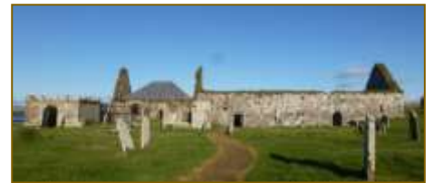
VIEW OF THE CONSERVED CHURCH WITH PROTECTIVE TEMPORARY ROOF OVER WEST CHAPEL TWO MAUSOLEUMS VISIBLE AT THE FRONT
