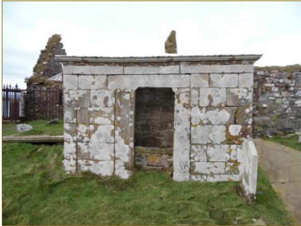
PROPOSED CONSERVATION OF EAST MAUSOLEUM WITH STONES REINSTATED (SOUTH ELEVATION ABOVE AND EAST ELEVATION BELOW)
