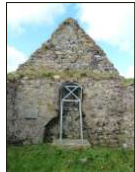
VIEW OF THE WEST GABLE OF WEST CHAPEL PRIOR TO PHASE 1 CONSERVATION – METAL SUPPORTING SYSTEM INSTALLED AROUND THE TIME OF UNDERPINNING WAS LATER REMOVED
