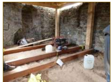
INSTALLATION OF TIE/STRUTS SYSTEM AT WEST CHAPEL
