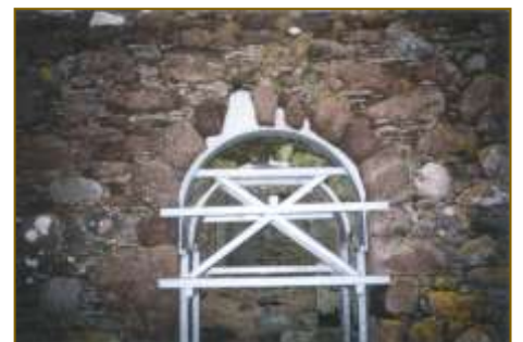
VIEW OF THE ARCHED DOORWAY BETWEEN THE CHURCH AND WEST CHAPEL AND ITS SUPPORTING SYSTEM
