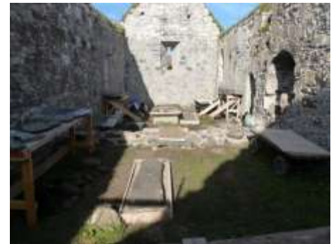
GRAVESLABS UNDER CONSERVATION
